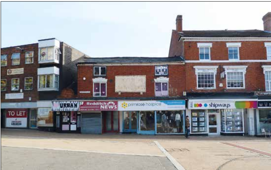
Oversized fascias and upvc windows to upper floors
