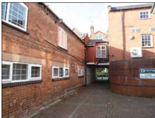
Rear of the entrance way which emerges onto Church Green between 10 and 12 Church Green East
